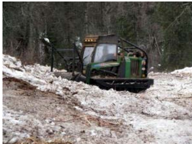
GyroTrac Working on the Hill Section.
